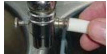
Attaching hose to diverter
