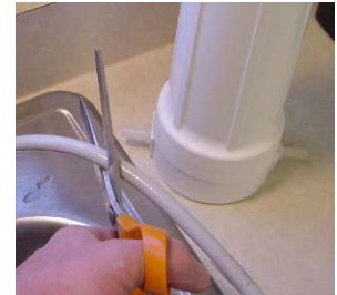
Cutting hose to length at optional prefilter
