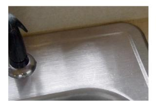
Identify suitable hole site - check for obstacles under sink.
