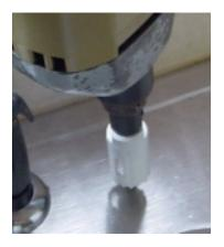
Carefully drill - do not force, you may have to reverse drill several times before penetration complete.
