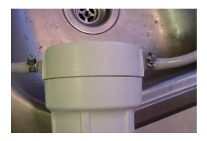
Identify prefilter input and output. Slide hose from saddle valve onto barbed fitting marked "Input" and secure with threaded clamp. Secure remaining hose end onto prefilter fitting marked "Output." Again, secure with threaded clamp.
