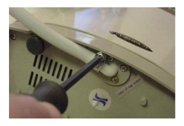
Press hose end from prefilter or saddle valve onto lon Farm water input and secure with threaded clamp.
