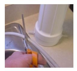
If installing Bluestone fluoride or carbon block prefilter, cut hose at the approximate installation location. Leave some slack for final positioning. If not installing prefilter, skip to step 17.
