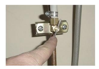
Open saddle valve by turning handle counterclockwise. Keep turning until you hear water flow. Inspect all connections for leaks and tighten clamps if necessary.
