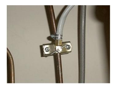
Press hose onto saddle valve barbed fitting and secure with threaded band clamp. Hose should press all the way onto fitting. (Hint: gently heat hose end with match or stove burner for easier placement.)
