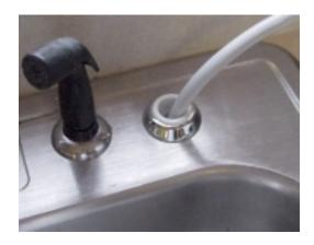
Feed hose end down through finished hole.
